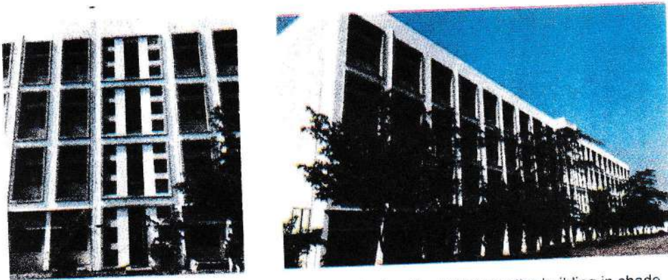
Projections in the form of fins and chajjas and vertical walls which keep the building in shade
