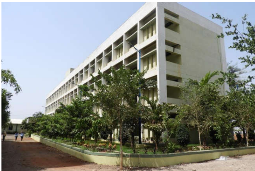
College Building – Side View
